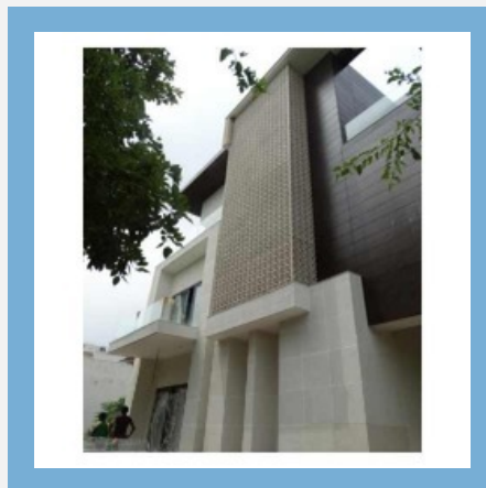
GRC Screens In Elevation
