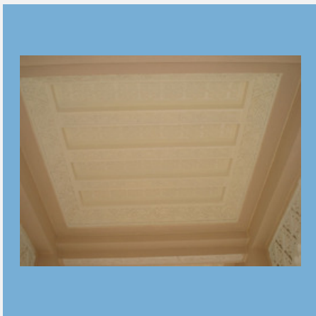
Decorative GRC Ceiling
