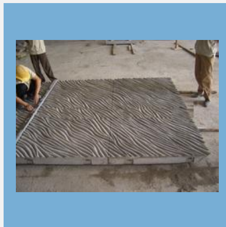
GRC Installation Services
