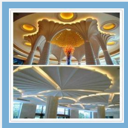
GRC False Ceilings
